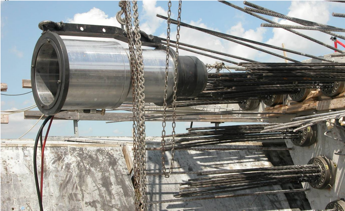
19G15 coupler under tensioning
